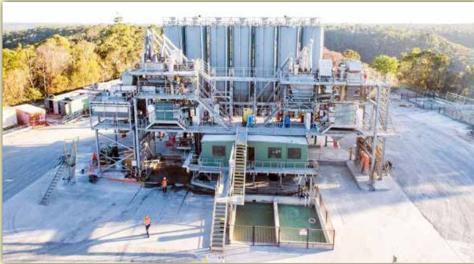
Copyright Boral. Image of larger facility at Mount Ku-Ring-gai.
