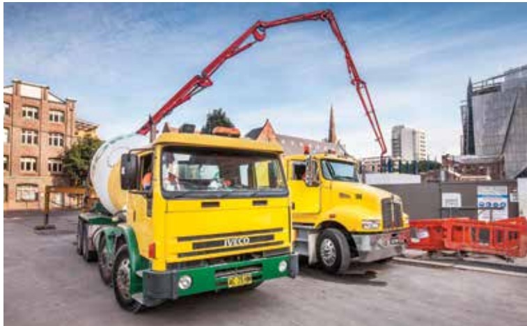
Boral Australia is seeking more regular use of its Glenorie concrete plant to support citywide building and construction
