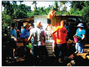
The earth-filled tubing walls rising and being compacted.
