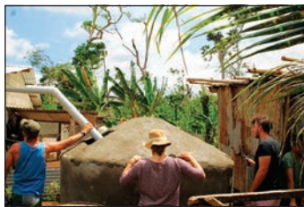
The final connection to the roof is being done – tank two in the outer suburbs of Vila.
