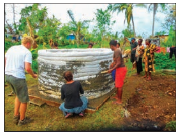
Students and the local women apply a cement render in order to protect the outside of the tank and make the inside watertight.
