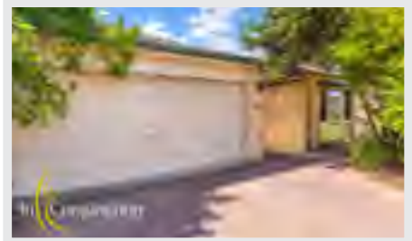
374B GALSTON ROAD, GALSTON
